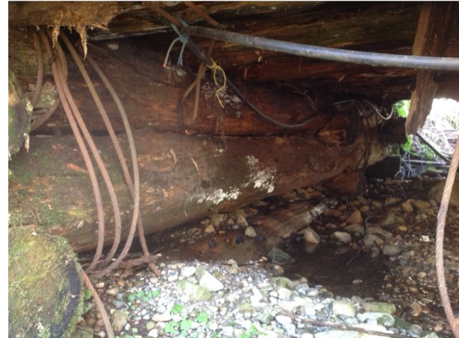
Right Bank Abutment when facing downstream
