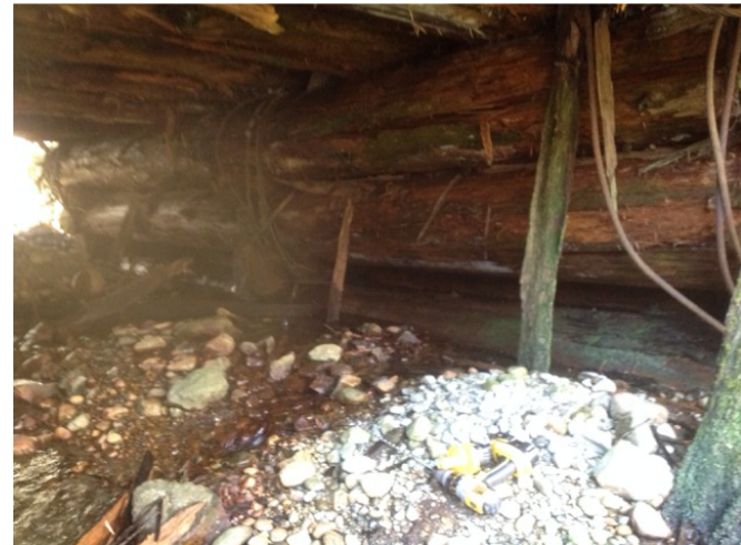
Left Bank Abutment when facing downstream
