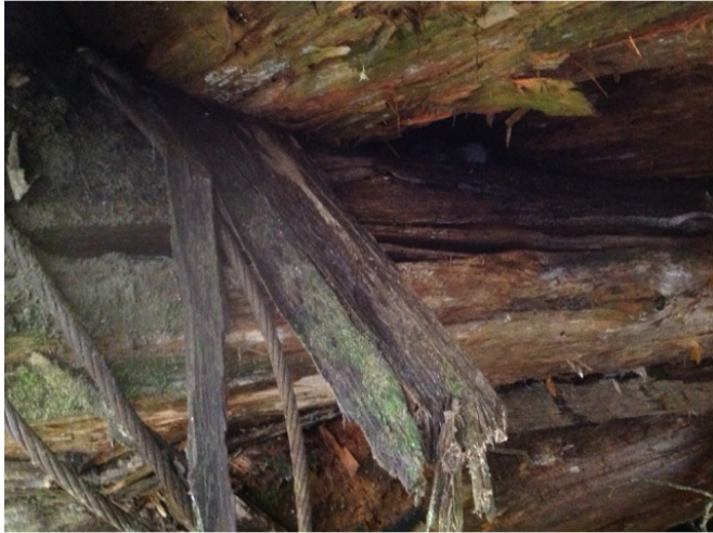
top crib log on left crib
